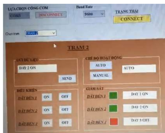
Figure 10. Control and monitoring application in computer.
